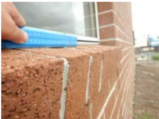
LHS- Step in bricks
