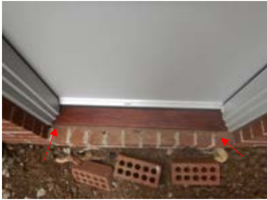
Out of square door tread with brickwork
