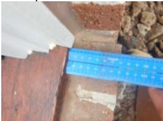
Out of square door tread with brickwork
