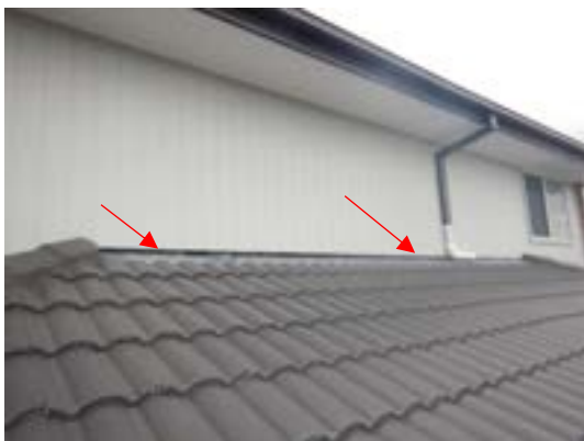
Flashing- Builder to clarify
