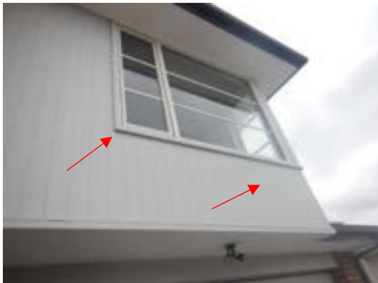
Chips and dents in cladding to a number of areas.
