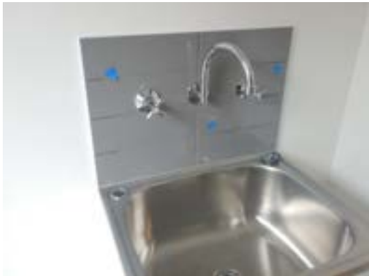
Colour variation in grouting
