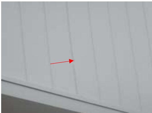
Chips and dents in cladding to a number of areas.
