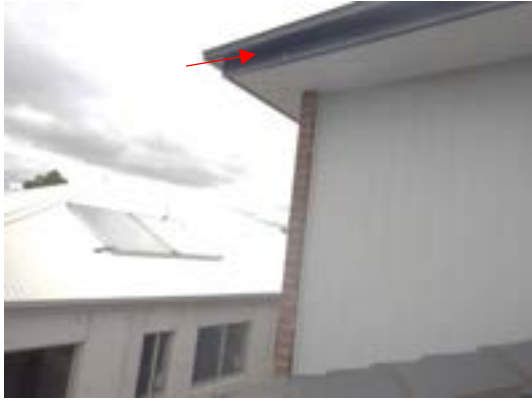
Fascia dent- Marked during previous inspection.
