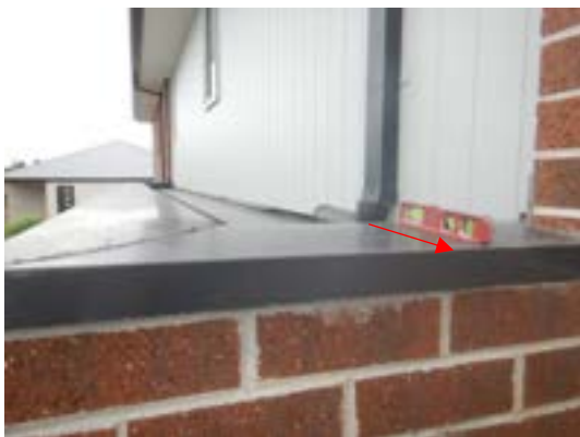
Flashing falling away from roof coverings
