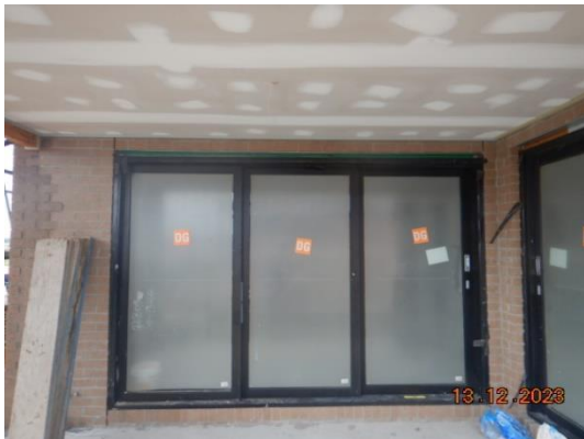
Quad out of parallel with bricks
