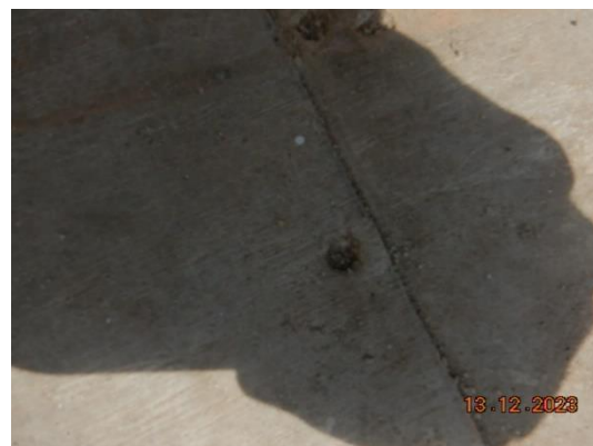
FIGURE 10 SEALING ALL JOINTS
