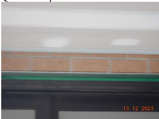
Quad out of parallel with bricks
