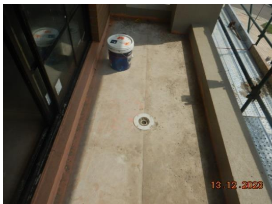
FIGURE 11 SEAL OVER FASTENERS AND JOINTS
