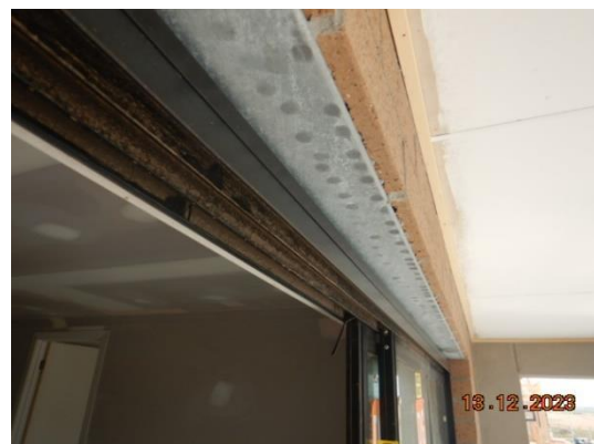
Discoloration spots to lintels
