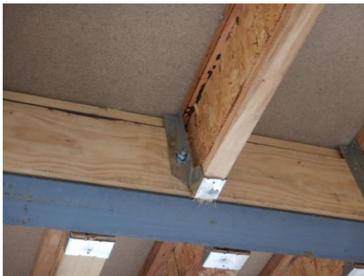
Damaged joist hangers due to bolt location
