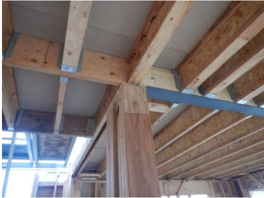
Complete joist hangers as per joist layout
