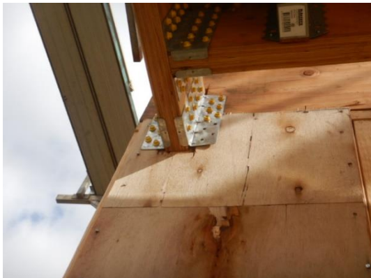
SPH220 require 10 screws to each face
