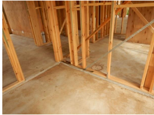
Rear internal garage wall
