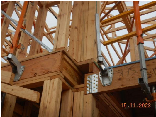
Figure 6.7 — Bottom plate stiffening
