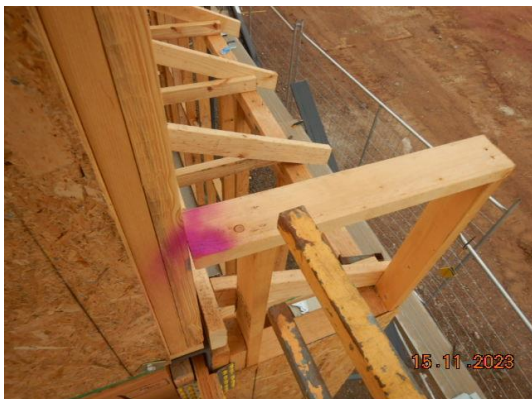
Secure parapet laterally
