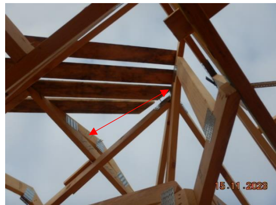
Ridge support block for valley boards
