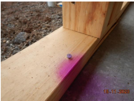
Ensure all masonry nails are hit home
