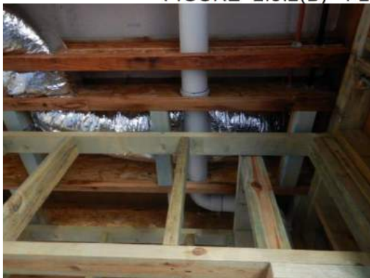
FIGURE 2.5.2(B) FLEXIBLE DUCT INSTALLATION
