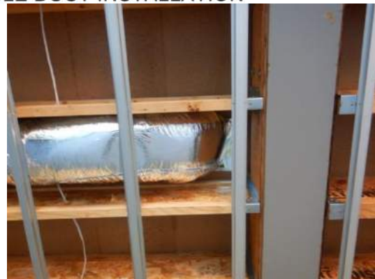
FIGURE 2.5.2(B) FLEXIBLE DUCT INSTALLATION
