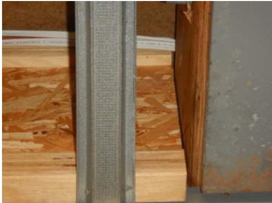
Missing joist hanger
