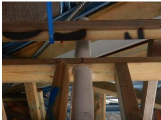
Stiffening to the plate required
