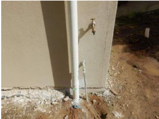
Drain under tap
