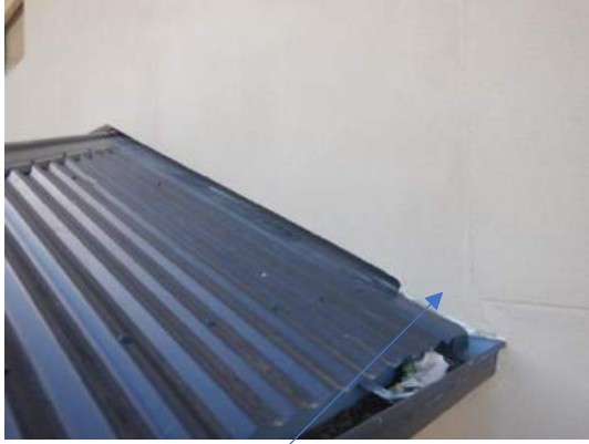
Missing Flashing
