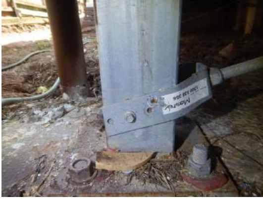
Brace to post one tech screw
