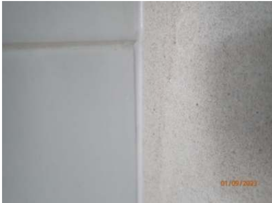
Tiles to internal corner cut short
