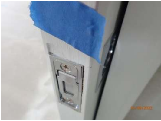
Rework plate installation - rough
