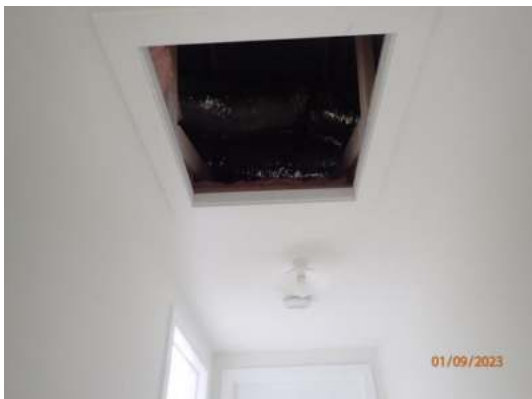
Install manhole cover
