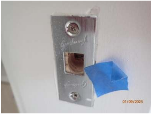
Rework plate installation
