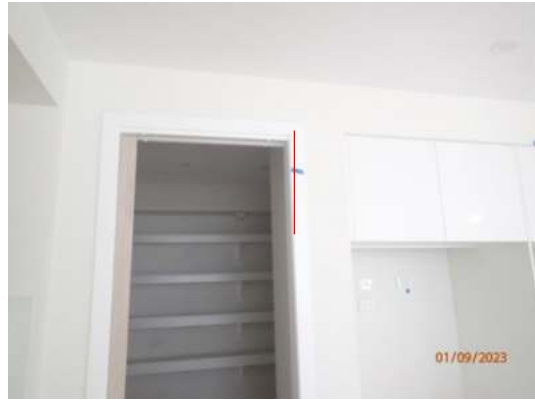
Arch out of plumb – top section
