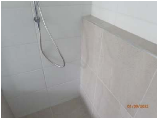
Tiles to internal corner cut short
