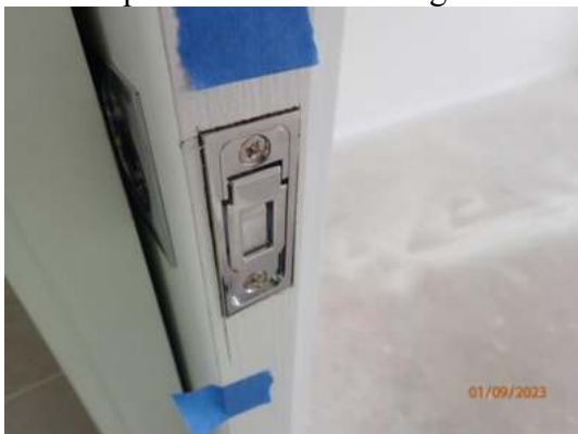
Rework plate installation - rough
