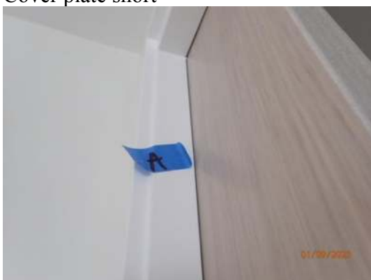
Adjust cavity slider margins
