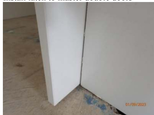
Install latch to master double doors
