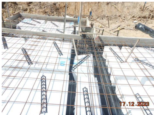
FIGURE 3.4 (in part) WAFFLE RAFT
