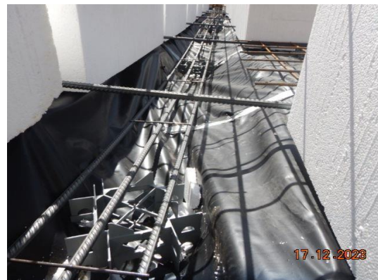
FIGURE 3.4 (in part) WAFFLE RAFT
