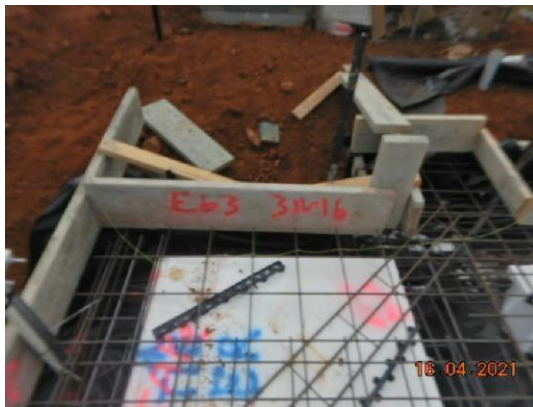
3-N16 Bars top & bottom to edge beam EB3
