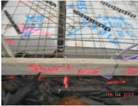
Short 1-N16 bar bottom internal rib
