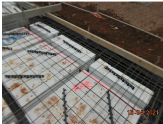
Missing N12 bar to internal top of rib
