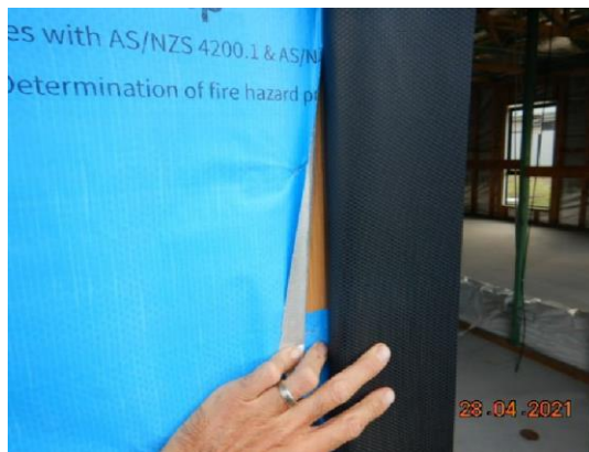
FIGURE 4.7 (in part) EXAMPLE OF WINDOW MEMBRANE TRIM DETAIL
