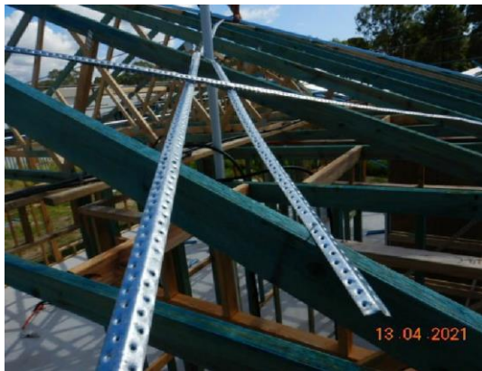
Bent around pipe and loose
