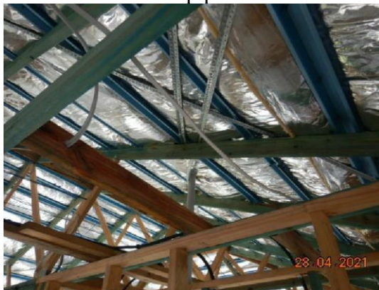
Bent around pipe and loose
