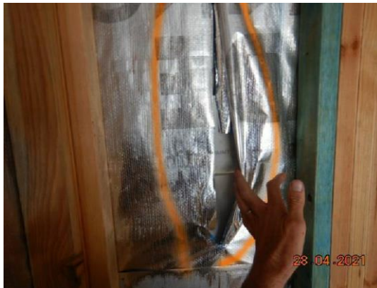
Tear in sarking sheeted over
