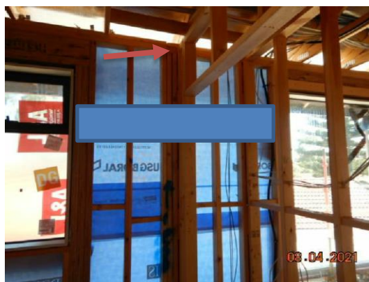
FIGURE 2.9 STUD/PLATE LAMINATION
