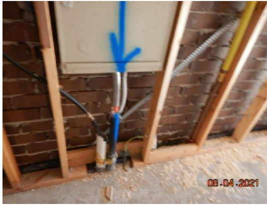
Pole protruding past frame
