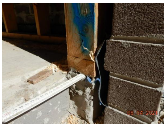
Gaps between frame and grout
