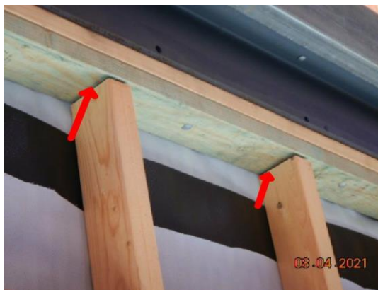
Short studs rear wall
