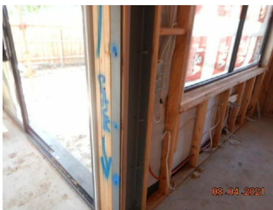
Bolt heads protruding past wall frame
