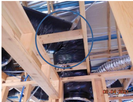
FIGURE 2.5.2(B) FLEXIBLE DUCT INSTALLATION
