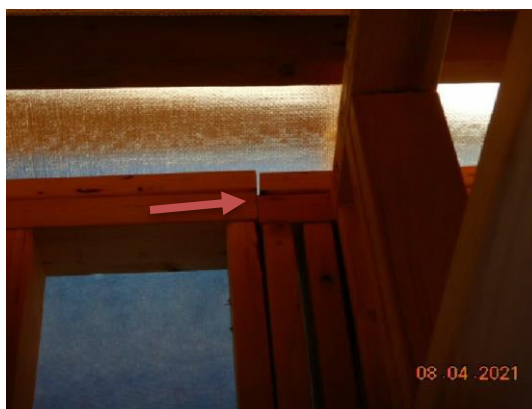
FIGURE 2.9 STUD/PLATE LAMINATION
