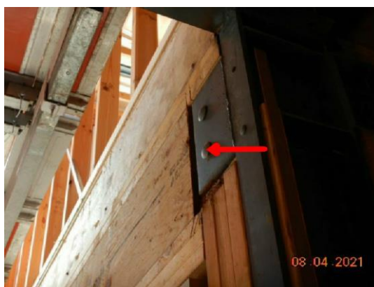
Short studs rear wall
