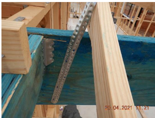
Extra nailing required, check all.
