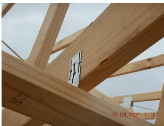
FIGURE 2.3 FIXING OF TRUSSES TO FREESTANDING NON-LOADBEARING WALL THAT IS NOT A BRACING WALL
