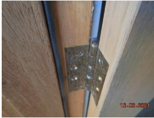
Discoloured hinges- most likely due to the acid the wash process.
