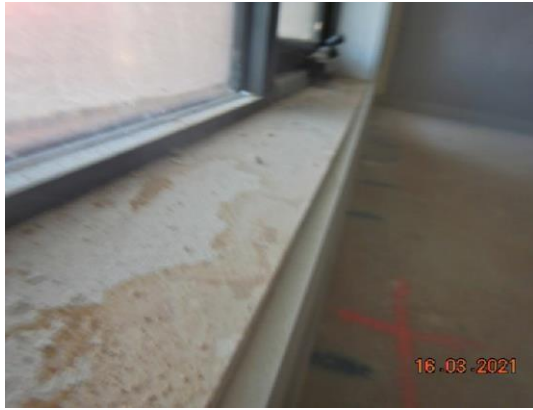
Water retention to a large number of MDF members.
