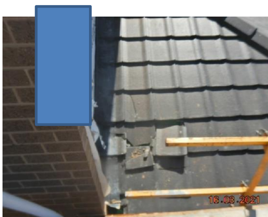
Large number of broken roof tiles
