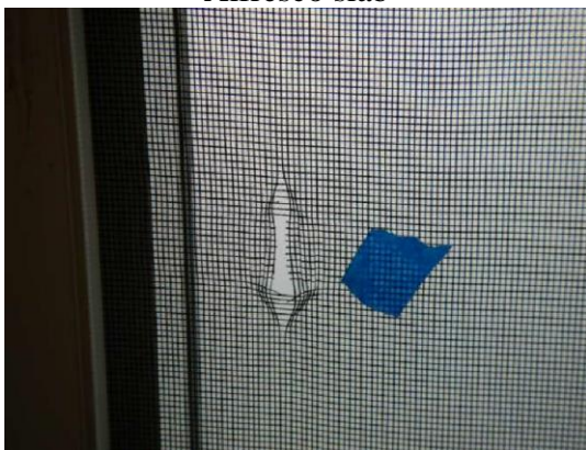
Damaged fly screen's multiple locations
