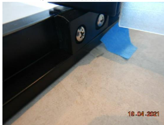
Wedge sticking out under screens
