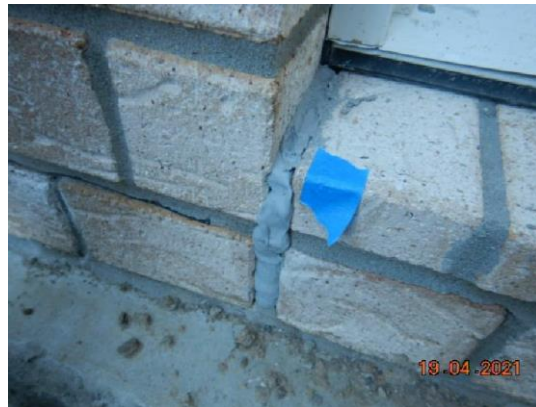
Silicone not tooled off
