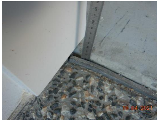
FIGURE 5.4.3 TYPICAL ISOLATION JOINT
