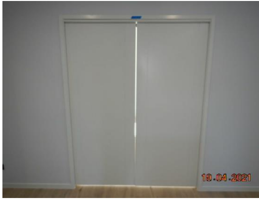
No door stops or handles fitted
