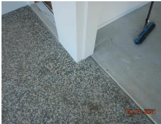
FIGURE 5.4.3 TYPICAL ISOLATION JOINT
