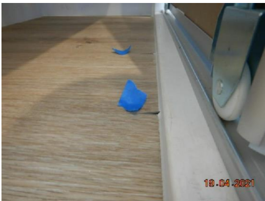
Areas of flooring rasied and not stuck down to slab.
