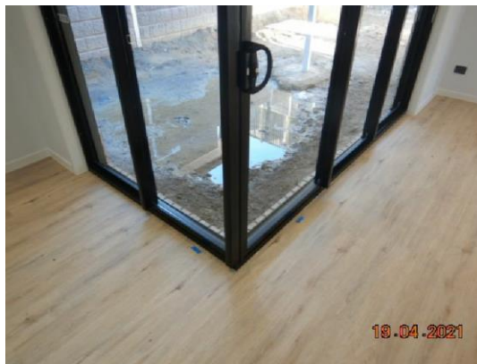
Areas of flooring rasied and not stuck down to slab.
