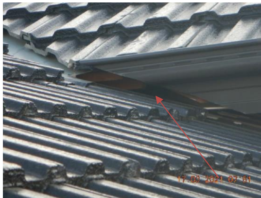
Excessive gap, rework.
