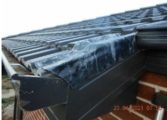
Unsightly flashing, poor workmanship.
