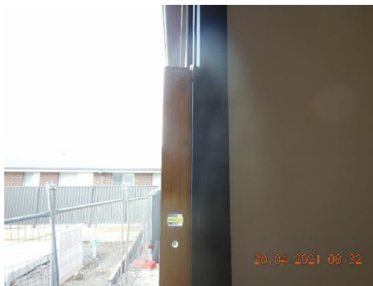
Frame is still bowed, door difficult to latch.
