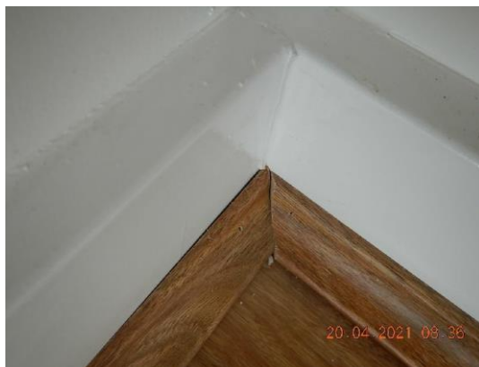
Out of alignment, all to comply.
