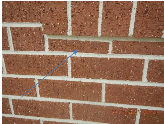
Brick OOL front elevation.
