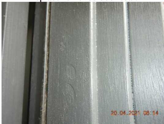
Hammer damage garage rear door.
