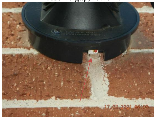
Excessive gap, rework.
