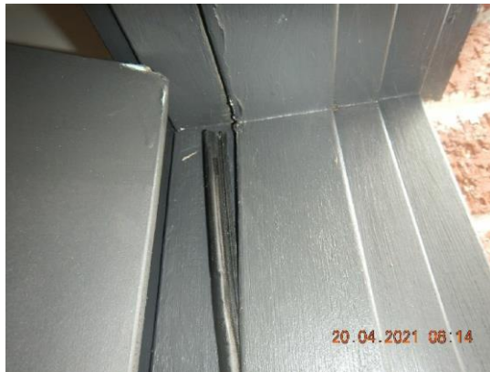
Damaged door seal.
