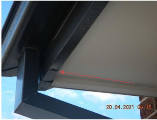
Dint, front elevation LHS.
