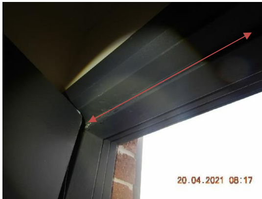
Replace removed door seal.
