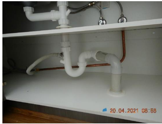
Exposed copper pipe not fixed.
